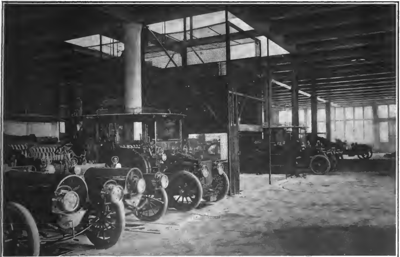
INTERIOR OF GARAGE PROPER OF NEW DECAUVILLE ESTABLISHMENT, SHOWING TWIN FREIGHT ELEVATORS WITH TURNTABLE IN FRONT.
